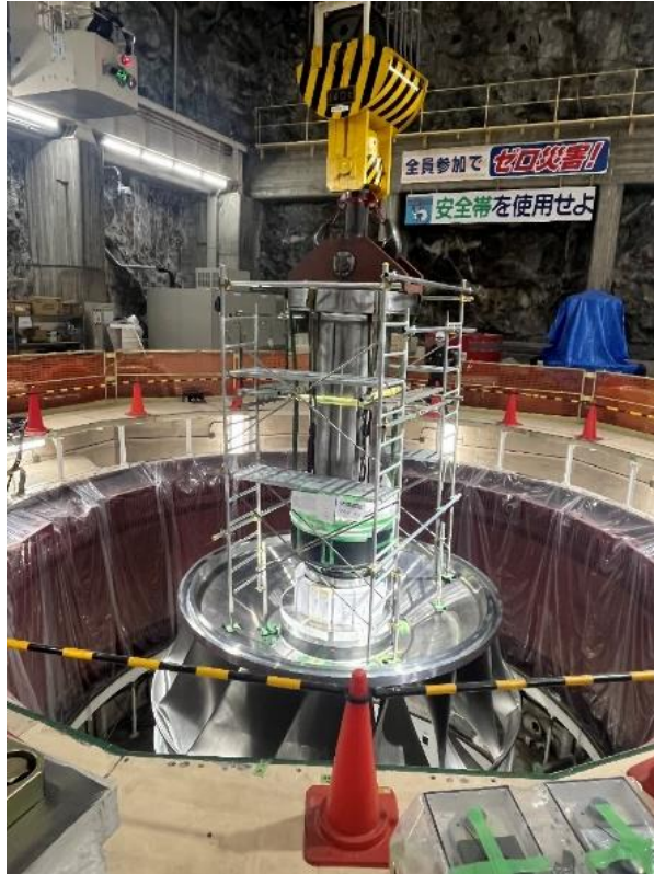
Installation of water turbine runner
