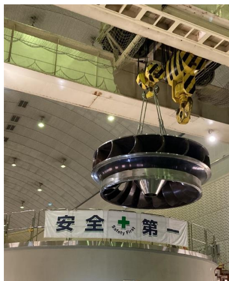
Installation of water turbine runner
