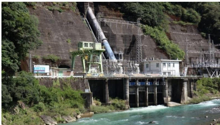
Nagayama Power Station (exterior view)
