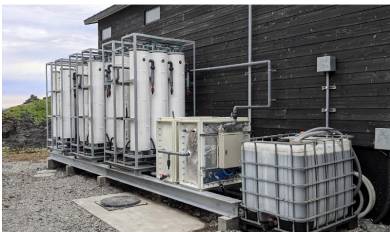
Photo: Watasumi's organic wastewater treatment system
