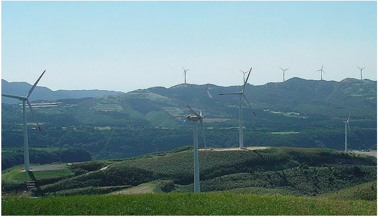
Minamiosumi Wind Farm (equipment before replacement; already removed)
