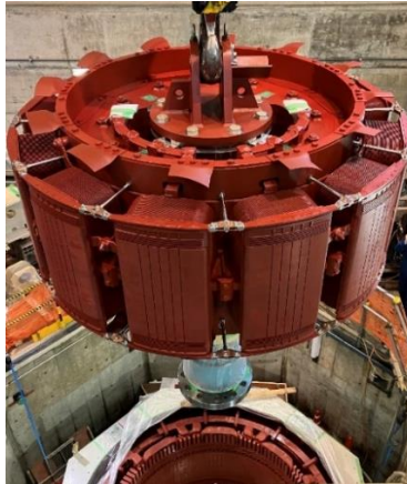
Ogamigo Hydroelectric Power Station (installing the new generator rotor)
