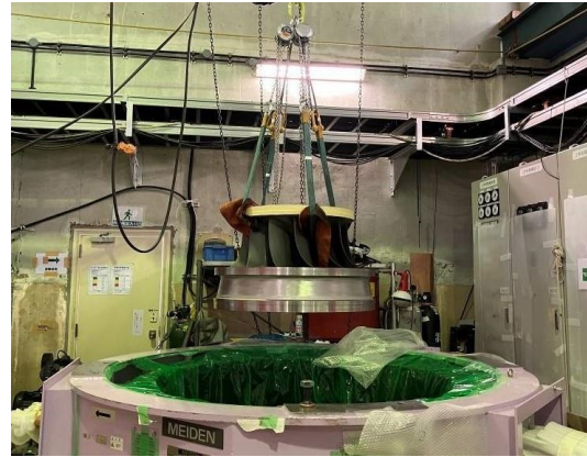
Installation of new water turbine runner for Unit 2
