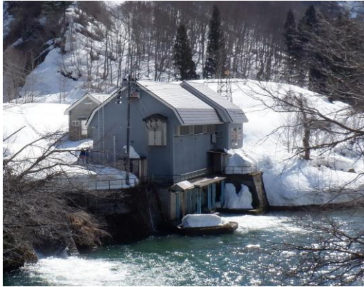
Suezawa Hydroelectric Power Station (full view)
