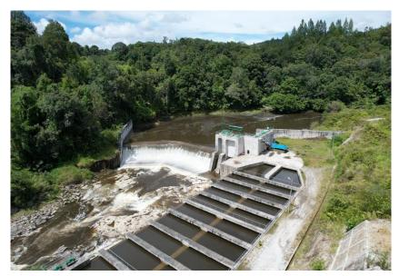
Sion Power Station: Weir and water intake
