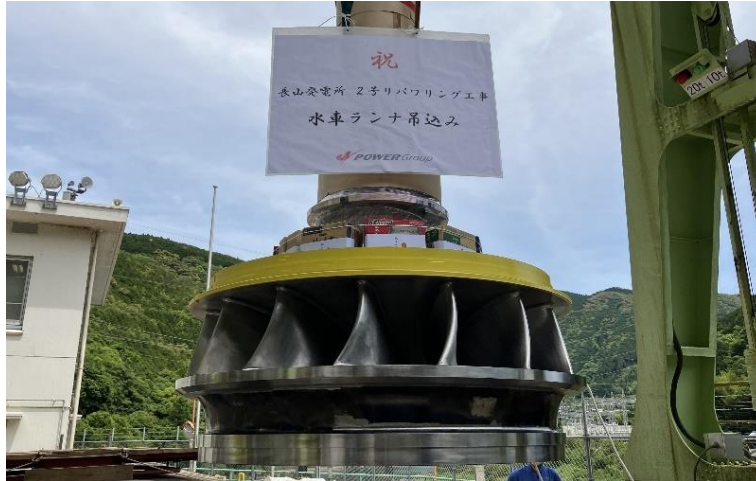
Nagayama Power Station Unit 2 during modernization (installation of water turbine runner)
