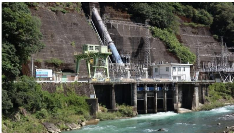
Nagayama Power Station (exterior view)
