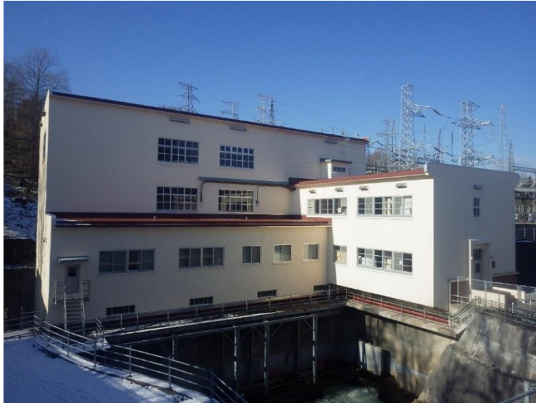
Ashoro Power Station (exterior view)
