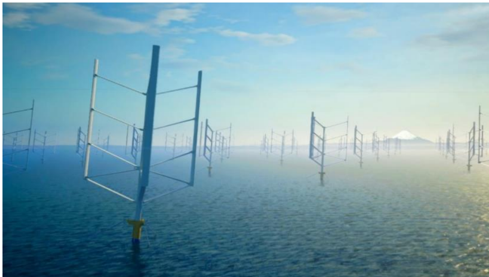
Image of a floating axis wind turbine (FAWT) wind farm
