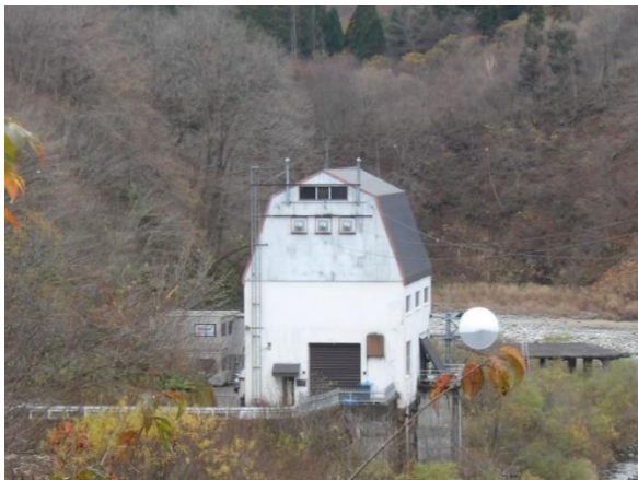
Exterior view of the power station
