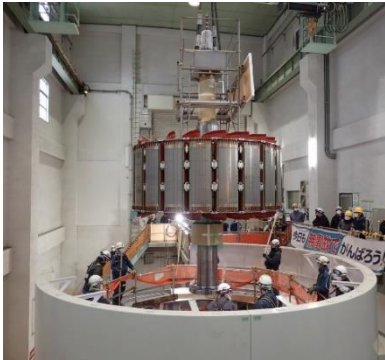
Installing rotor (December 2022)
