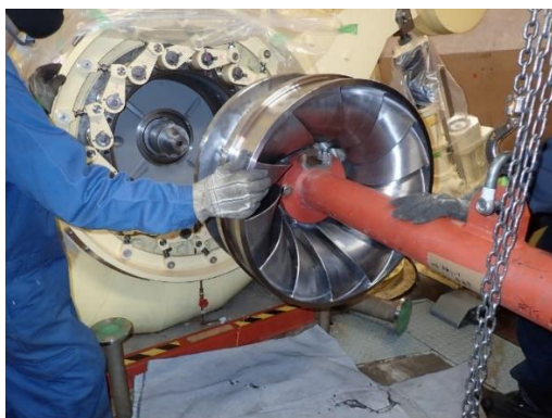
Installation of new water turbine (Tagokura Hydroelectric Power Plant)
