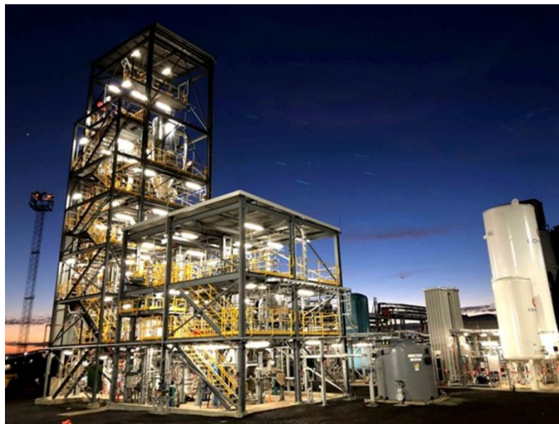
Figure 2. Coal gasifier and hydrogen refining facility
