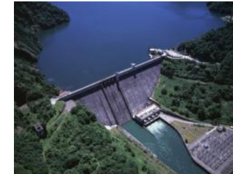
Tagokura Power Plant
