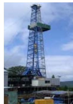
[Exploratory Well Drilling]
