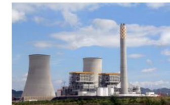
Henzou Power Plant (China)
