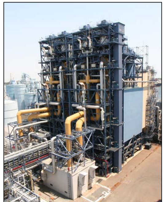
ReACT (J-POWER Isogo New No. 2 Thermal Power Station)
