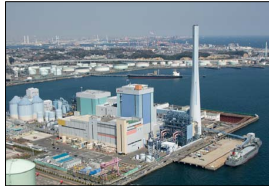
Isogo Thermal Power Station New No. 2 Unit (left) and New No. 1 Unit
