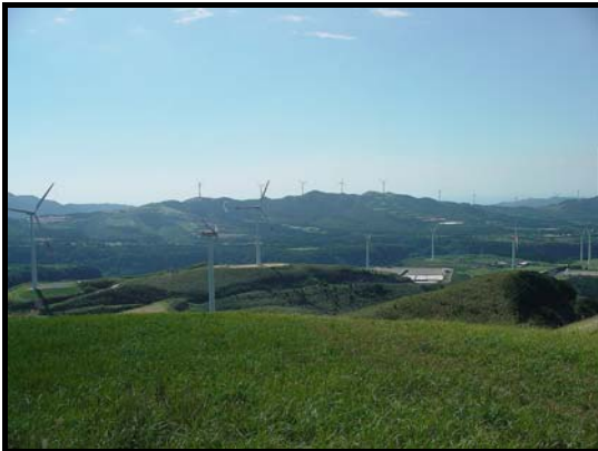
Minami Oosumi Wind Farm (Minami Oosumi-cho, Kimotsuki-gun, Kagoshima Prefecture)
