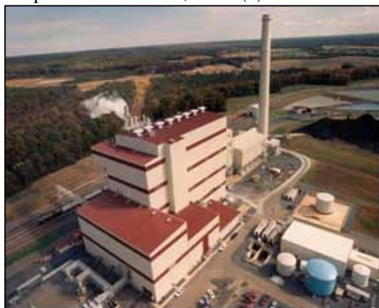
Birchwood Power Station
