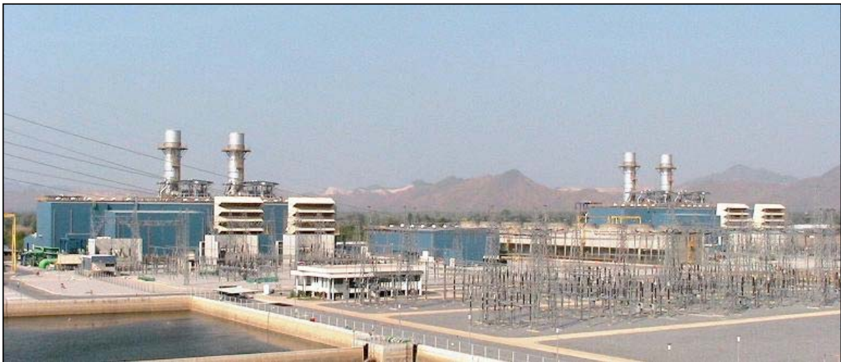
Kaeng Khoi #2 Power Station (Block 1 to the left, Block 2 to the right)
