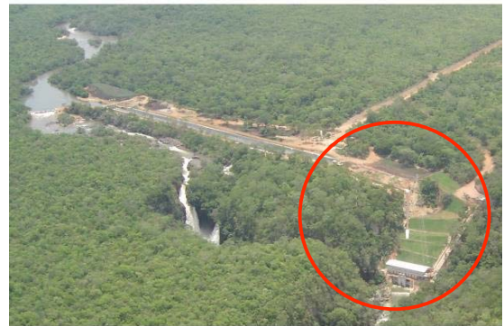
Aquarius Hydroelectric Power Plant
