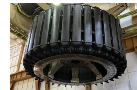
Lifting Out the Generator Rotor of Unit1
