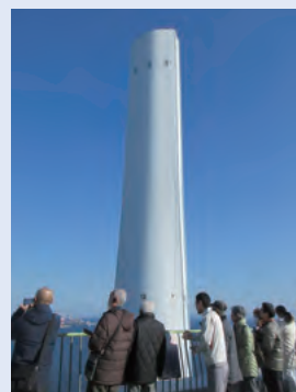
Facility tour for shareholders (Chimney at Isogo Thermal Power Plant)
