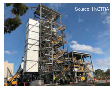
Brown coal gasification furnace facilities under construction
