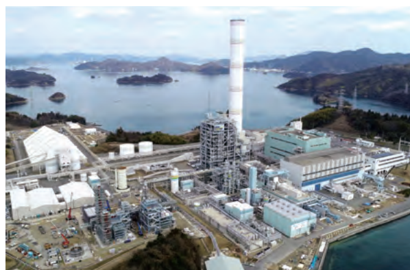
Osaki CoolGen Project demonstration test facilities (Osakikamijima-cho, Hiroshima Prefecture)
