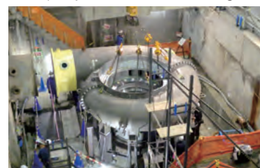
Construction on the Shinkatsurazawa Project
