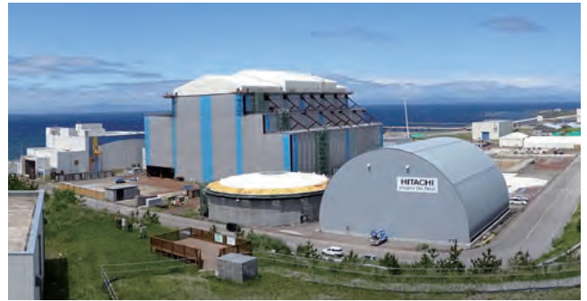
The Ohma Nuclear Power Plant under construction (June 2020)
