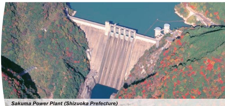
Sakuma Power Plant (Shizuoka Prefecture)
