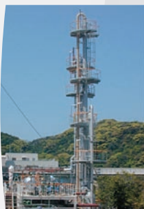
Facility for demonstrating CO 2 separation and recovery at the Matsushima Thermal Plant, Unit 2
