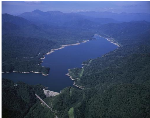
Nukabira Dam (Hokkaido prefecture)
