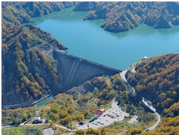
Okutadami Dam (Fukushima prefecture, Niigata prefecture)
