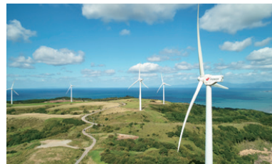
Kaminokuni Wind Farm
