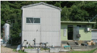
Decentralized water supply (Ishima small-scale water supply)
