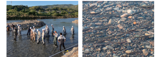
Leveling gravel on the riverbed
