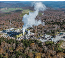
Appi Geothermal Power Plant
