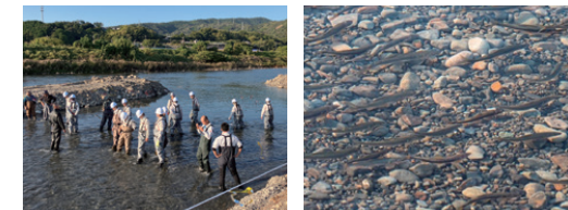
Leveling gravel on the riverbed
