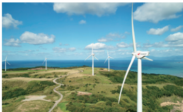
Kaminokuni Wind Farm
