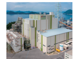
Takehara Thermal Power Plant
