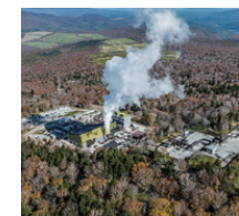
Appi Geothermal Power Plant
