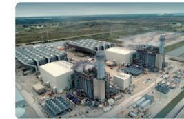
Jackson Thermal Power Plant (Commercial operation began in 2022)
