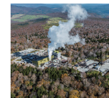
Appi Geothermal Power Plant
