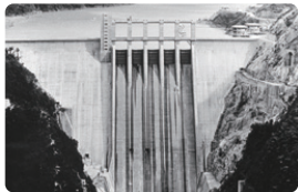
Sakuma Dam (Completed in 1956)
