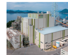
Takehara Thermal Power Plant
