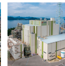
Takehara Thermal Power Plant New Unit No. 1
