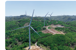
Kaminokuni No. 2 Wind Farm, Hokkaido Owned capacity: 41.532 MW
