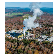
Appi Geothermal Power Plant
