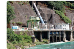
Nagayama Hydroelectric Power Plant Unit 2, Kochi Pref. Owned capacity: 18.5→19.25 MW (750 kW increase by repowering)
