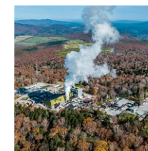
Appi Geothermal Power Plant
