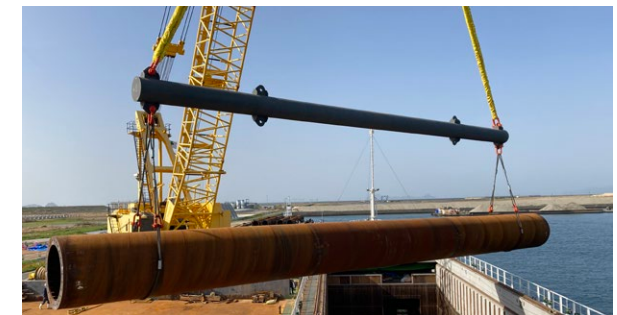
Pile delivery for wind turbine base
