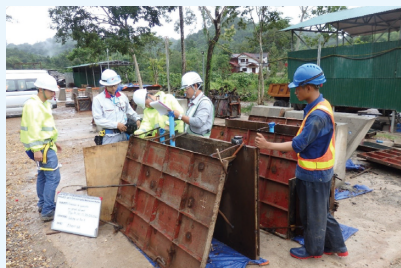
Inspecting shuttering for concrete
