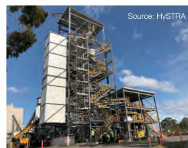
Brown coal gasification furnace facilities under construction
