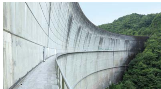
Ikehara Power Plant (Nara Prefecture)
