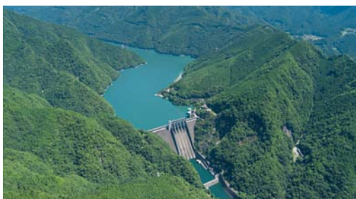
Sakuma Power Plant (Shizuoka Prefecture)
