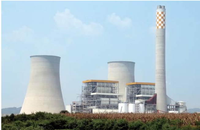
Hezhou Power Plant (China)
