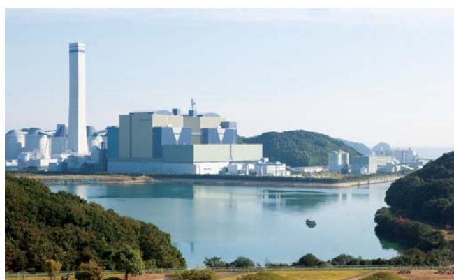
Tachibanawan Thermal Power Plant
