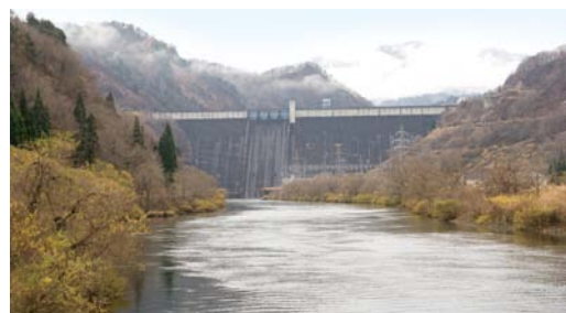
Tagokura Power Plant (Fukushima Prefecture)
