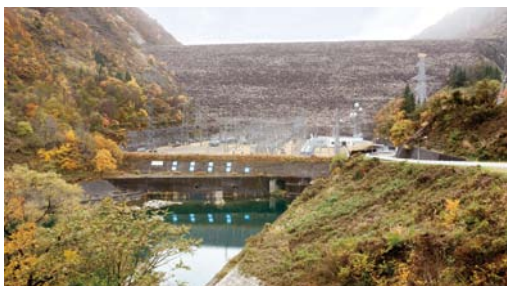
Miboro Power Plant (Gifu Prefecture)
