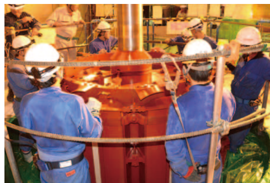
A view of the generator (rotator) suspended (Isawa Hydroelectric Power Station, Iwate Prefecture)
