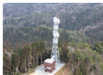
Tsuge Radio Relay Station (Nara Prefecture) A microwave radio relay station that links power stations, transformer stations, and other facilities. The station is highly reliable in order to ensure uninterrupted communications even in the event of a disaster such as an earthquake or typhoon.
