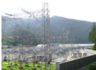
Sakuma Frequency Converter Station (Shizuoka Prefecture) This converter station enables the transmission of electricity between the different frequencies of eastern Japan (50 Hz) and western Japan (60 Hz). It is the world's first electricity business frequency converter station built to support efficient electric power operations.
