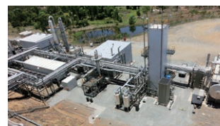
Exhaust gases containing high concentrations of CO 2 are condensed and cooled to capture liquid CO 2 of a high degree of purity
