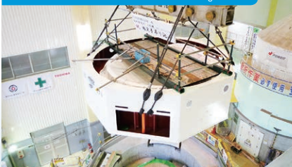
Nukabira Power Station Unit No. 2 stator being lifted in
