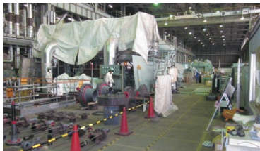
No. 1 Unit undergoing periodic inspection (forefront is No. 1 Unit steam turbine)
