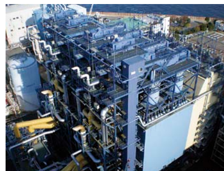
Dry-Type Desulfurization-Denitrification facility for J-POWER Isogo Thermal Power Station
