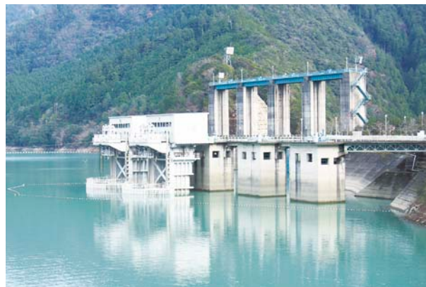
Surface-water intake equipment (Ikehara Dam, Nara Prefecture)
