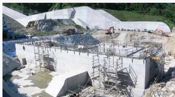
Status of Pouring of Foundation Concrete for Power Station (Taken May 2012)
