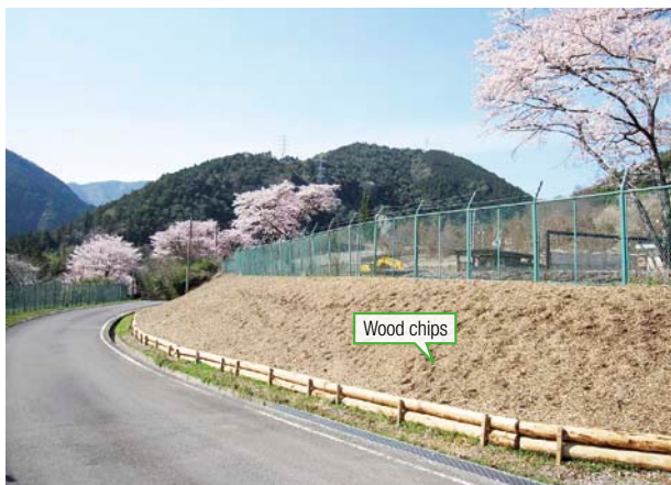
Wood chips used as ground cover (Nanairo Power Station, Wakayama Prefecture)
