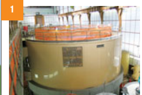
Sakuma No. 3 Unit being overhauled
