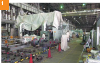
No. 1 Unit undergoing periodic inspection (forefront is No. 1 Unit steam turbine)
