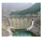
River maintenance flow discharge (Itoshiro Dam, Fukui Prefecture)
