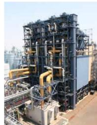
Dry-type desulfurization system at Isogo Thermal Power Station new No. 2 unit (Yokohama)
