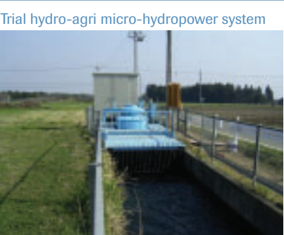
J-POWER co-developed a hydro-agri micro-hydropower system, which makes effective use of the utilized head of water in existing irrigation channels, and commercialized it after conducting trials in fiscal 2004. <System Overview> Power generation method: Waterfall Effective head of water: 2m Maximum capacity: 30kW
