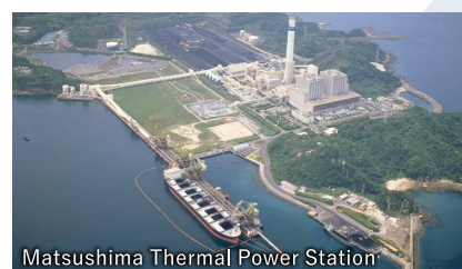
Matsushima Thermal Power Station
