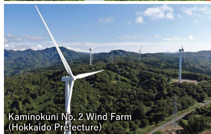
Kaminokuni No. 2 Wind Farm (at the time of construction)
