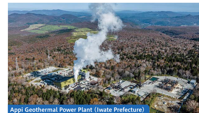
Appi Geothermal Power Plant (Iwate Prefecture)
