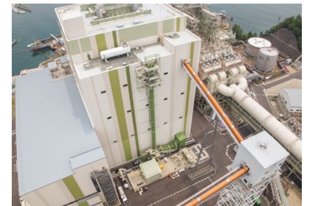
Takehara Thermal Power Station New Unit No. 1 (Hiroshima Prefecture)
