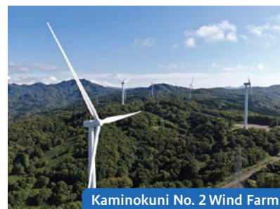
Kaminokuni No. 2 Wind Farm
